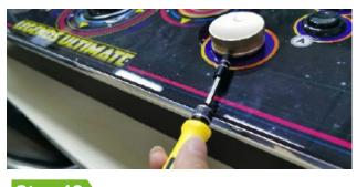
**Step 13** Fasten the spinner cap with the hex key.
